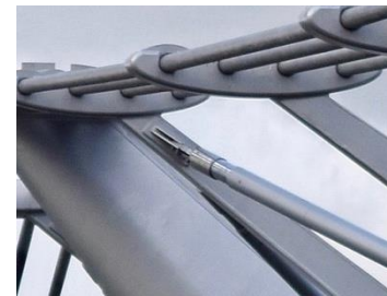
Moving end of pier damper
