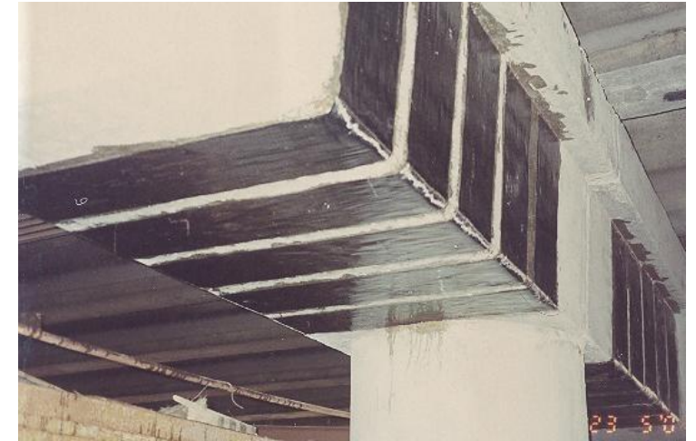
Shear strengthening
