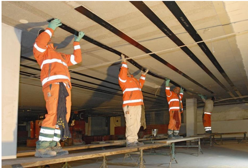
Flexural strengthening
