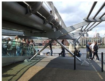
Vertical to ground dampers
